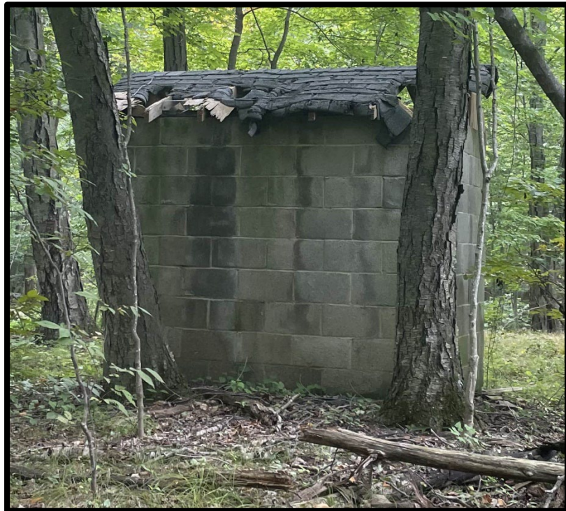
A - 4 Rear view of outhouse structure.
